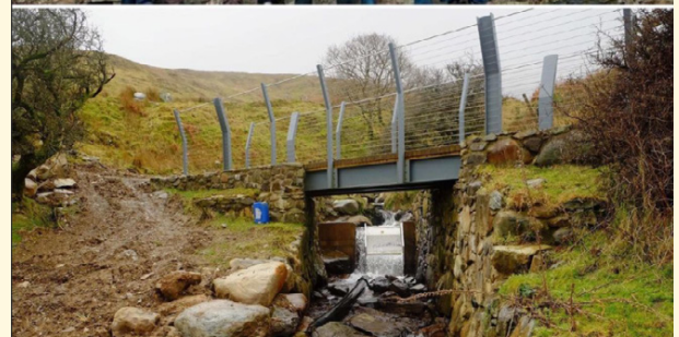
Top: Cyd Ynni Members, bottom: Hydro Installation
