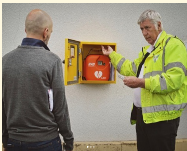
Gwent Energy CIC's local installed defibrillator
