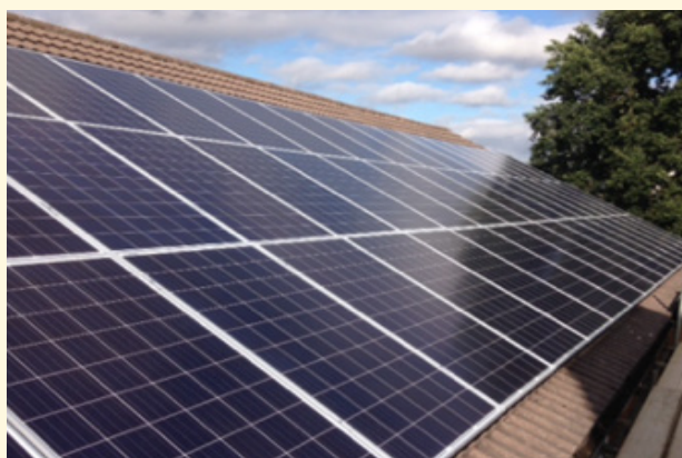
Solar Installation by Harborough Energy
